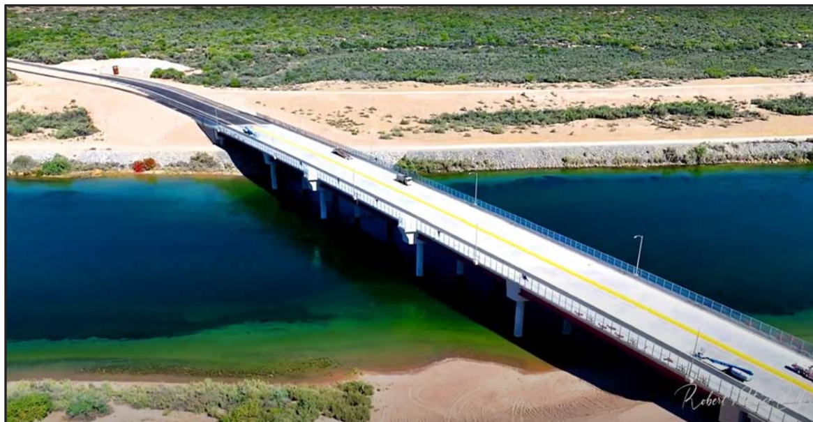
Aerial Image of the Laughlin-Bullhead City bridge. Set to open on June 7, 2024, the bridge promises to enhance connectivity and foster economic growth for the communities on both sides. (Image courtesy of Robert Bilbray via YouTube.)
